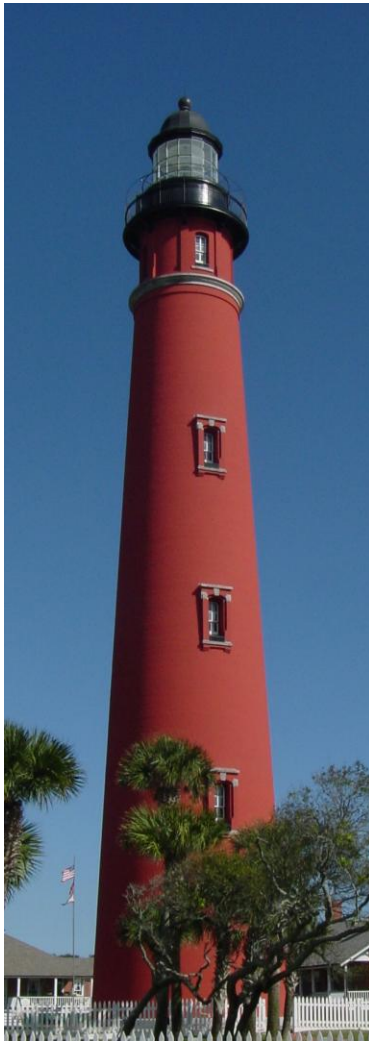
Ponce de Leon Inlet Lighthouse
