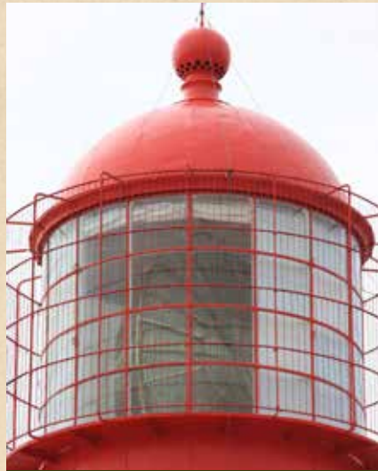
The lighthouse's distinctive Red Lantern room houses a rare 1st order hyper-radiant Fresnel Lens.
