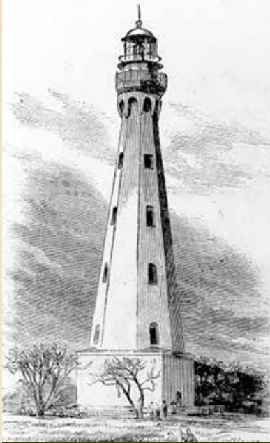
Rebuilt in 1789, the second Charleston Lighthouse was octagonal in shape and originally utilized a spider lamp as its beacon. Source: www.wikimedia.com
