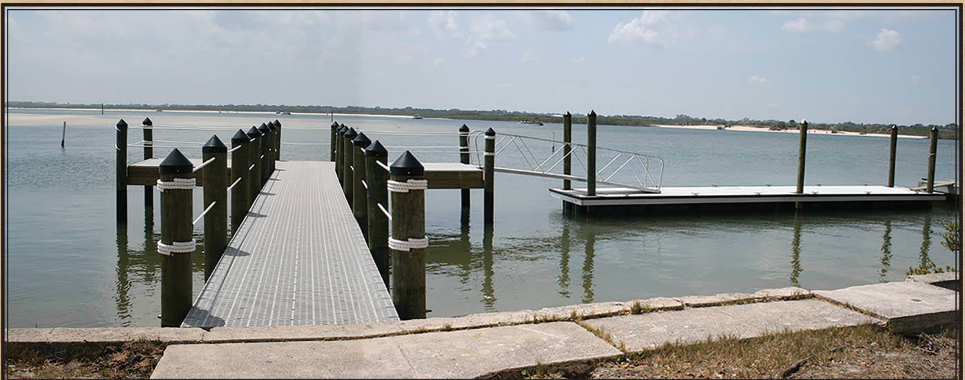
The new Pacetti Hotel dock occupies the same footprint as its predecessor with the addition of a new floating dock section.
