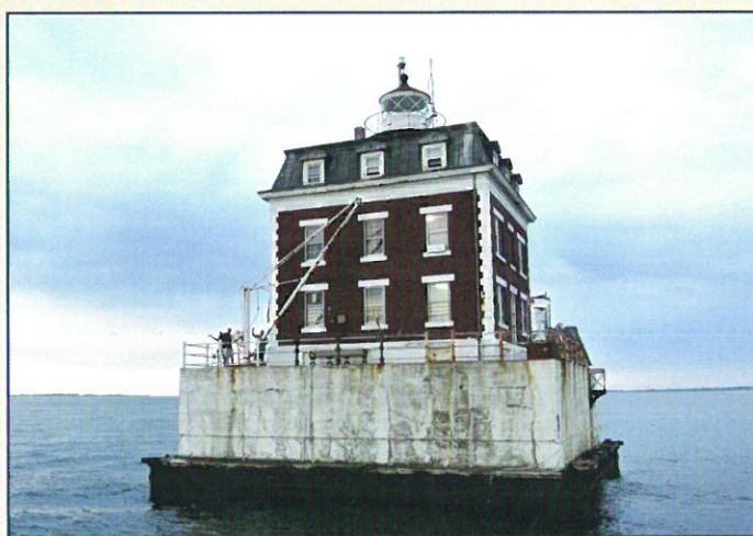
Perched atop a concrete pier situated at the mouth of the Thames River in Fishers Island Sound, the New London Ledge Lighthouse is a 58-foot structure of unique design. Borrowing from both the Colonial Revival and French Second Empire architectural styles, this three story brick and granite lighthouse was completed in 1909 to guide ship transiting Connecticut’s New London Harbor. Operating as a harbor light, the required range of the lighthouse’s beacon was nominal, resulting in its relatively low if not elegant stature.
